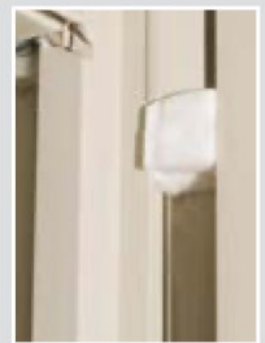
Foam blocks reduce air infiltration.
